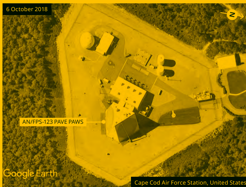
FIGURE 16-31 – CAPE COD MISSILE WARNING RADAR
