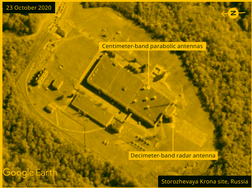
FIGURE 16-48 – KRONA RADAR COMPLEX NEAR STOROZHEVAYA
