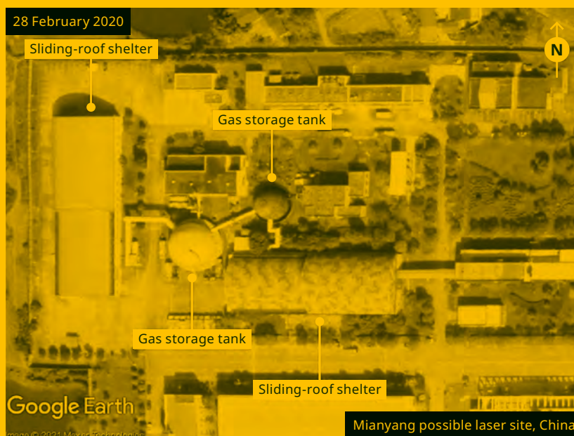
FIGURE 16-29 – LASER TEST SITE NEAR MIANYANG
