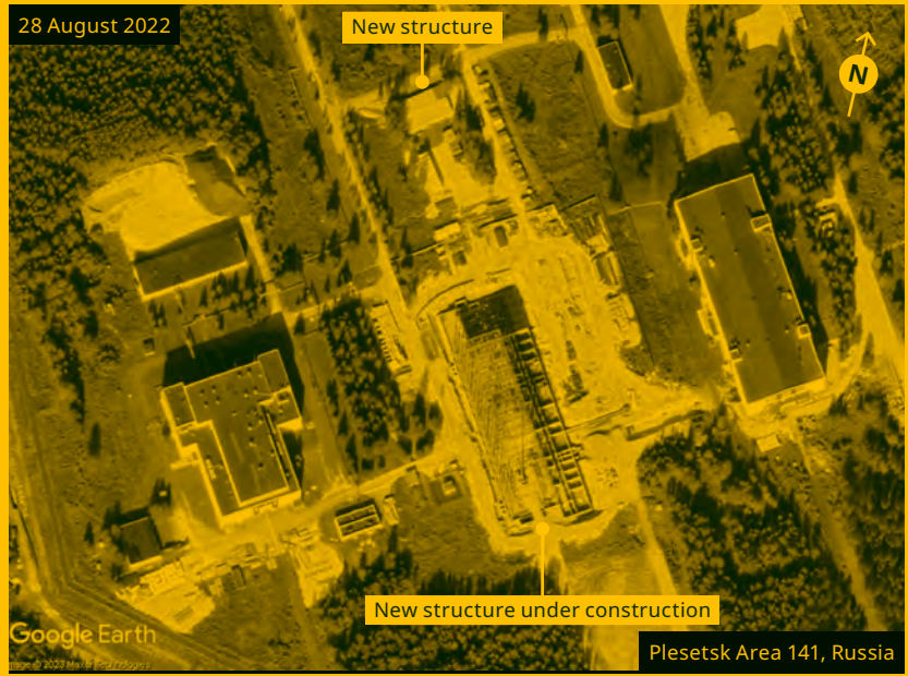
FIGURE 16-8 – PLESETSK AREA 141 BUREVESTNIK FACILITIES
