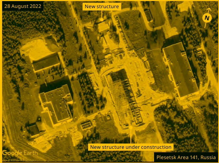
FIGURE 16-8 – PLESETSK AREA 141 BUREVESTNIK FACILITIES
