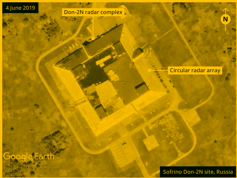
FIGURE 16-45 – DON-2N SITE AT SOFRINO
