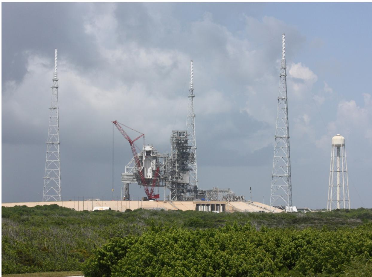
**Figure 4. Lightning masts at Pad 39B. Image credit Wikimedia Commons ([source](#)).**
