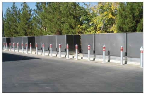
Figure 4-16: 800 kW SOFC system outside a Walmart [Bloom Energy, 2010].
