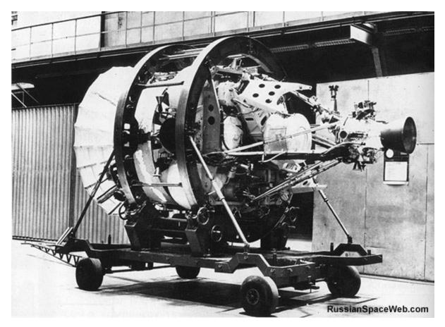
Figure 17. Photo of the Soviet IS killer satellite during ground processing. Image courtesy of the <u>Russianspaceweb.com</u> Credit: TsNII Kometa
