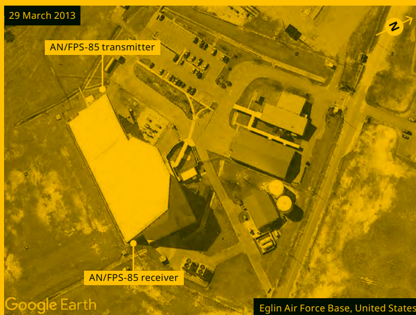
FIGURE 16-33 – EGLIN SPACE SURVEILLANCE RADAR
