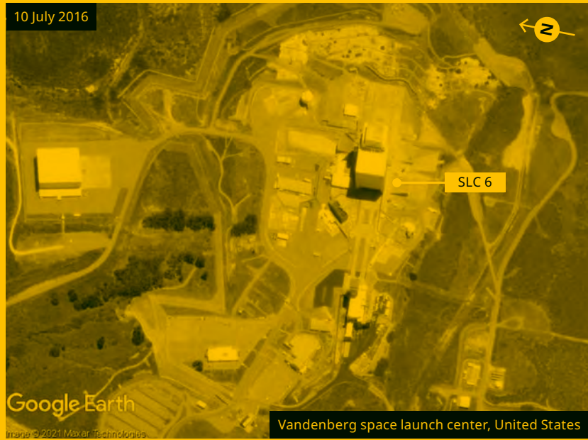
FIGURE 16-2 – VANDENBERG SPACE LAUNCH COMPLEX 6
