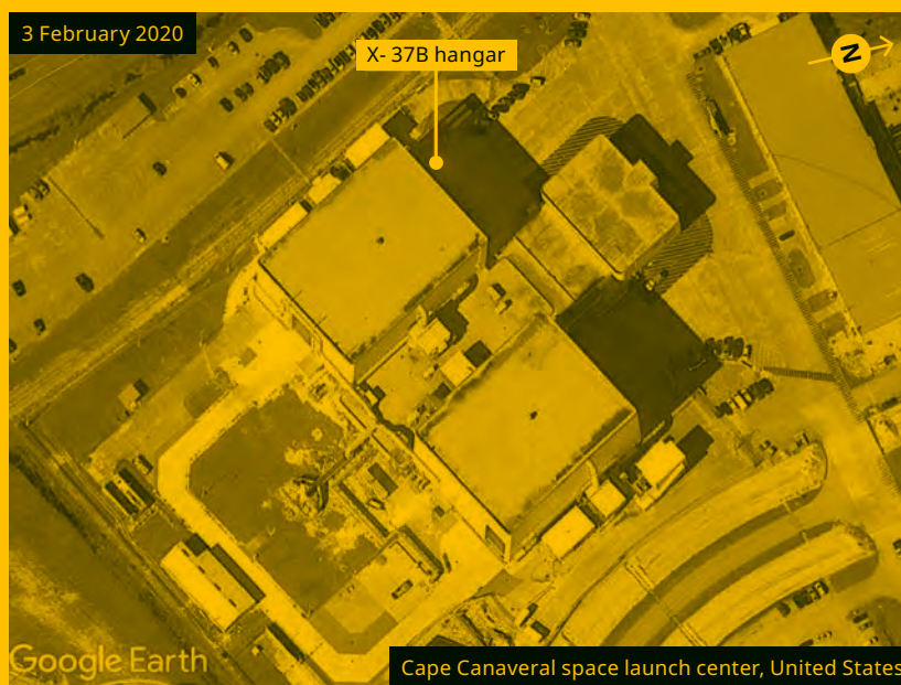
FIGURE 16-3 – CAPE CANAVERAL X-37B HANGAR
