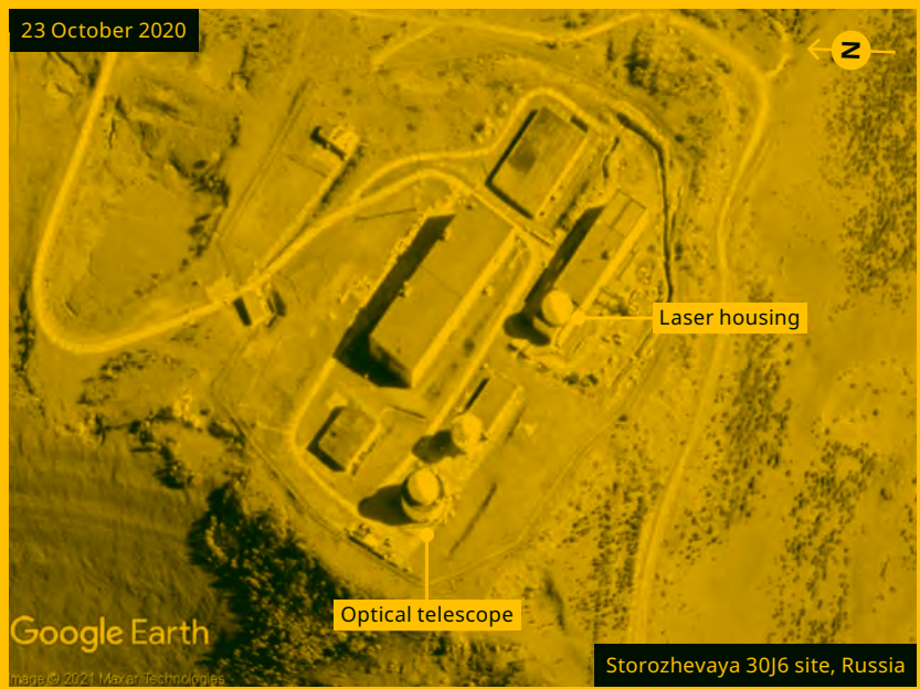
FIGURE 16-49 – KRONA 30J6 OPTICAL COMPLEX NEAR STOROZHEVAYA
