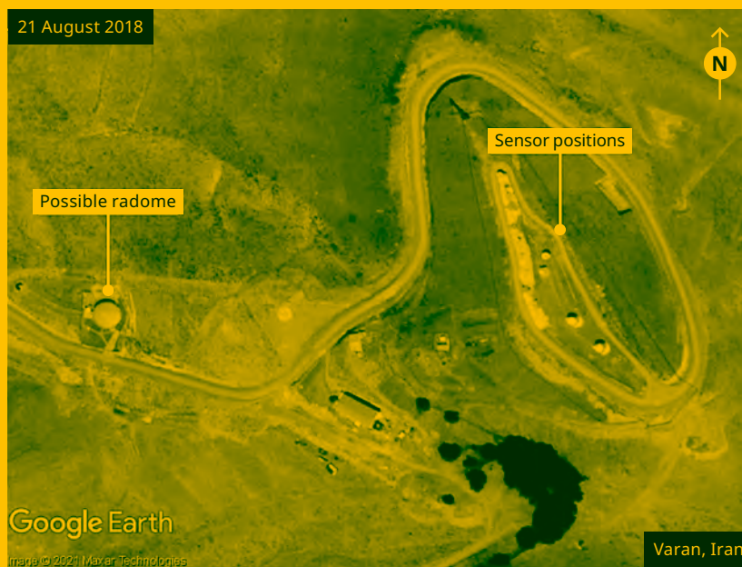
FIGURE 53 – DELIJAN SPACE TRACKING CENTER
