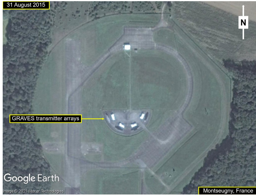
FIGURE 44 – GRAVES RADAR TRANSMITTER
