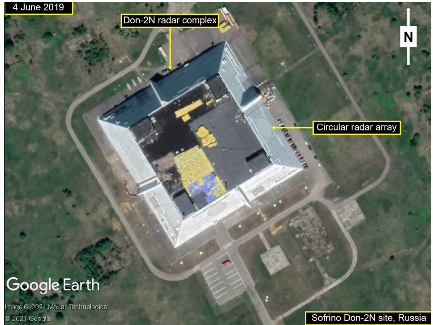
FIGURE 31 – DON-2N SITE AT SOFRINO
